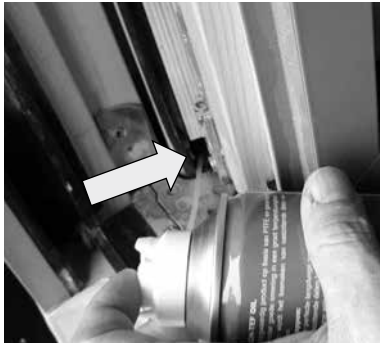
Lubricate the bearing point between the sliding surfaces with high-quality lubricant (e.g. Teflon oil).
