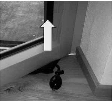
Lift the opened sash e.g. with an air wedge packer until the lower bearing point bears no weight.
