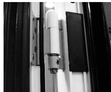
Remove the bottom cover caps.
