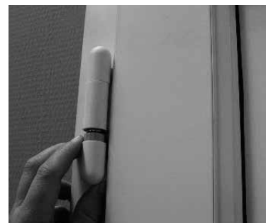
Remove the bottom cover caps.
